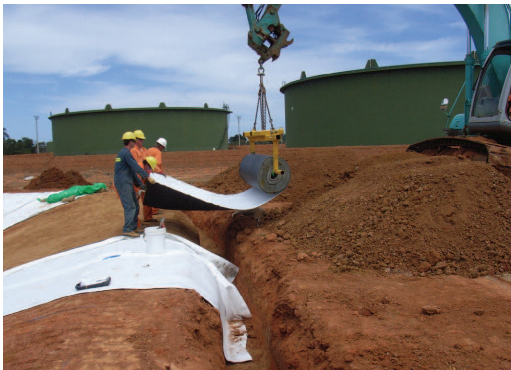
Installation of the Rawmat HDB lining system
